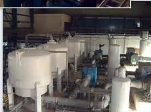
Gold Mine in Kazakhstan Two ASV33000 (868 Nm 3 /hr) Plants
